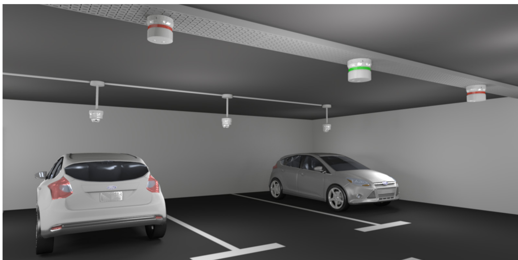
Fig. 4 One SBPILED indicator associated to each SBPSUSL sensor
